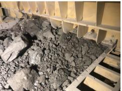
Forefront Services was engaged to carry out repairs to the lower front area of a ROM bin brow. The parent metal had worn away and required significant in situ repairs. The proposed repairs included cutting out the plate and gusset sections then fabricating sections on site for welding back into place. This method of repair meant many hours of cutting then fabrication and welding in the replacement sections. All of this carried out in the underground environment.
